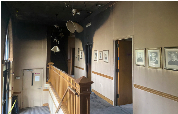
Deans’ Hallway showing fire damage (left) and following cleaning and sealing for access to the elevator (right)
